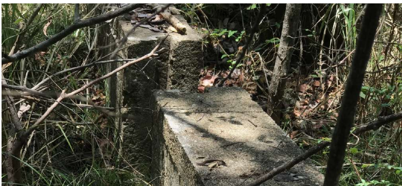
An abandoned sluice gate
